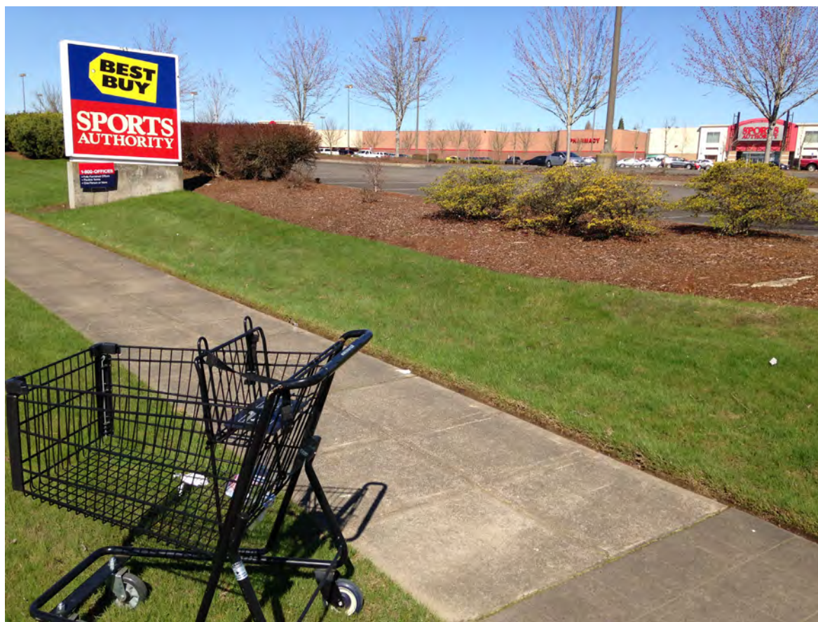
Commercial retail is single-story and automobile-dependent, separated from the adjacent streets by large parking lots.
