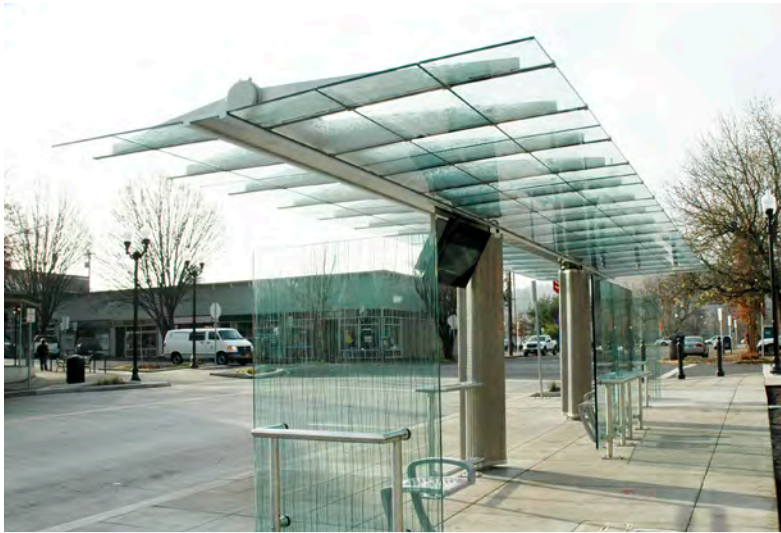
Enhanced transit shelter provides safe refuge from the elements and timely transit information
