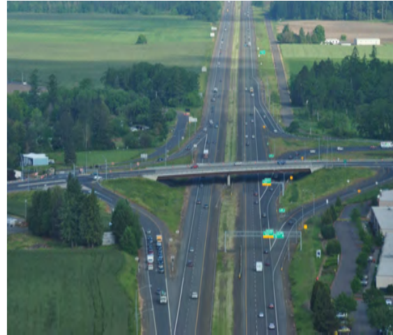
US Hwy 26 / NE Brookwood Interchange
