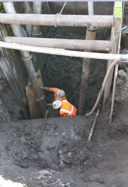
A Hillsboro Water Department employee goes underground to investigate a leak.
