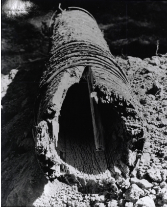
Hillsboro's wooden water pipe delivered to residents in 1913.
