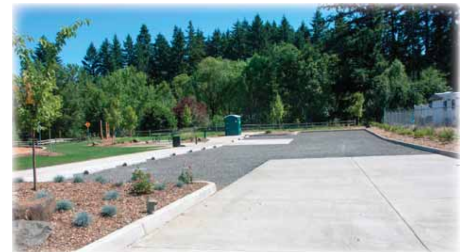
Cherry Lane Trailhead on the Rock Creek Regional Trail. An example of a small pervious gravel parking lot with concrete drive.
