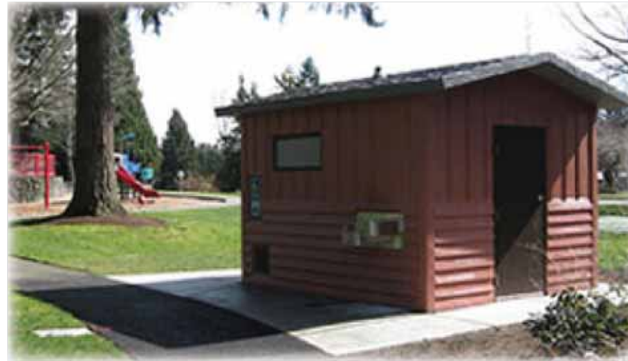
Single-stall prefabricated restroom
