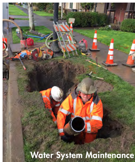
Fire Hydrant Installation
