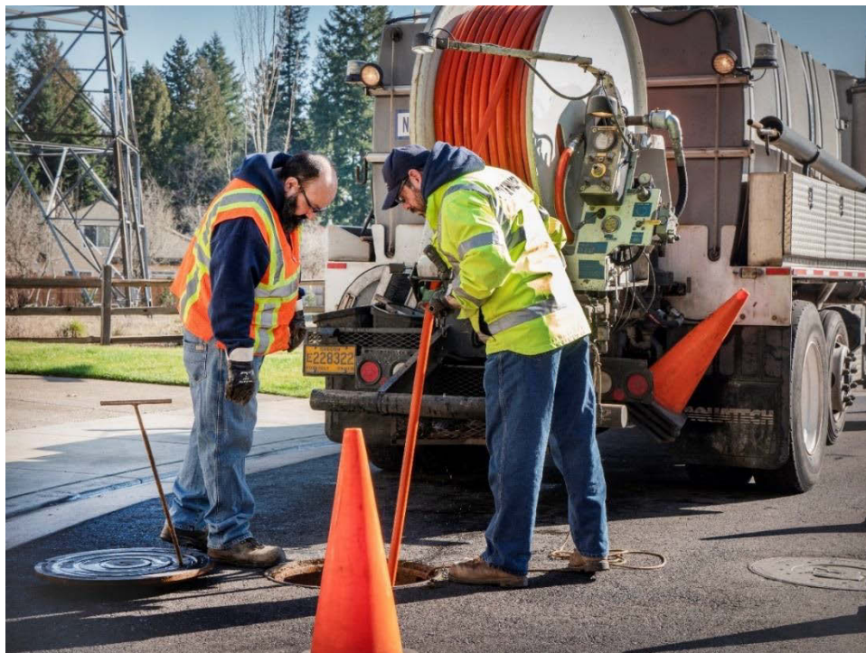
Figure 5-1. City maintenance staff using vacuum truck to clean sewer pipelines
