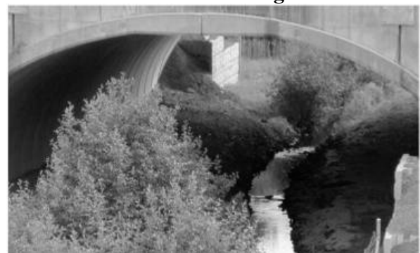
Figure 12.50.930-A: Examples of Stream Crossings with Fish and Terrestrial Wildlife Passage Provided
